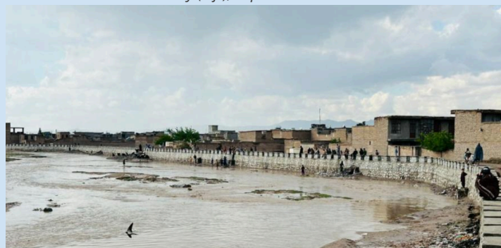
Flood protection wall in District 10 of Herat city, April 2026
