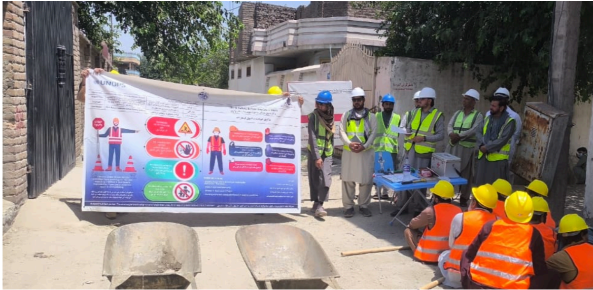
E&S awareness signboard - C2 project site - Jalalabad, June 2026
