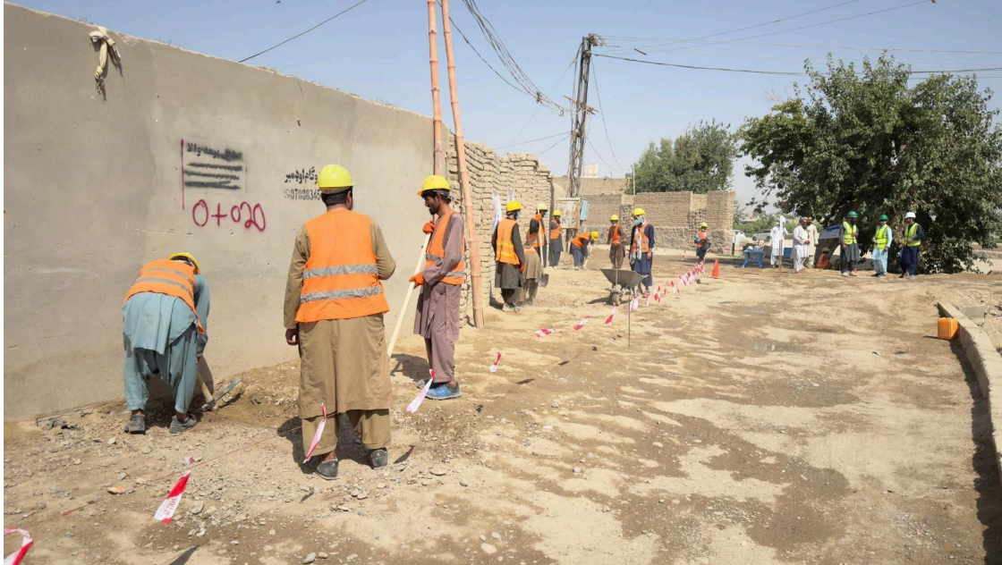
Excavation of roadbed in Sadat Qalachah Plum Concrete Streets, in Gozar 6 of District 3 of Kandahar City in June 2026 @UNOPS
