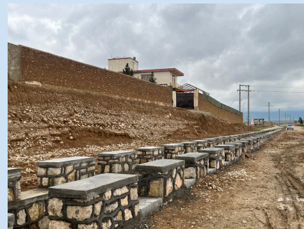
Construction of Kaj-Gozar Protection wall for Canal with total length 300 m, Gozar#15, District#11, Mazar-e-Sharif City (right) and Nahr-e-Babayadgar Stone Masonry Retaining Walls with total length of 550 m in Gozar#08, District#4, Mazar-e-Sharif City (left), September 2025
