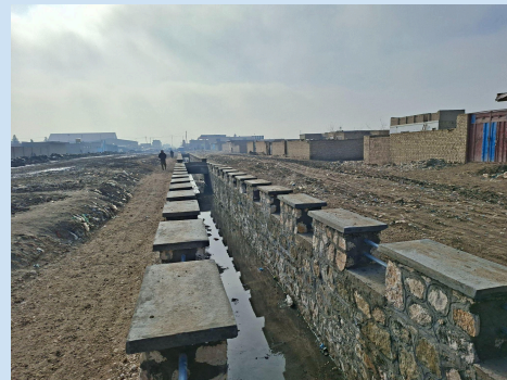
Construction of 2nd Dawlatabad protection wall Lot#1 for wastewater Canal with total length of 400 m, District#09, Mazar-e-Sharif City, April 2026
