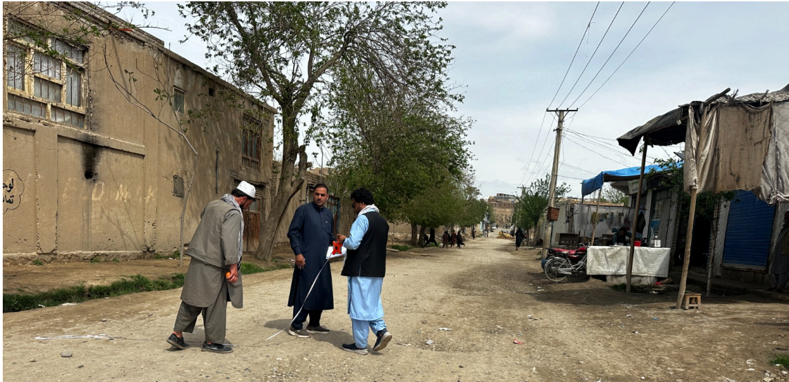
UNOPS Construction Management Engineer scoping a gravel surface road at Koti Gerd (L=540m), in Guzar 14 of District 3 of Kunduz City, April 2026 @UNOPS
