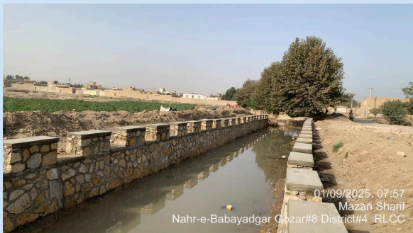
Construction of Kaj-Gozar Protection wall for Canal with total length 300 m, Gozar#15, District#11, Mazar-e-Sharif City (right) and Nahr-e-Babayadgar Stone Masonry Retaining Walls with total length of 550 m in Gozar#08, District#4, Mazar-e-Sharif City (left), September 2025
