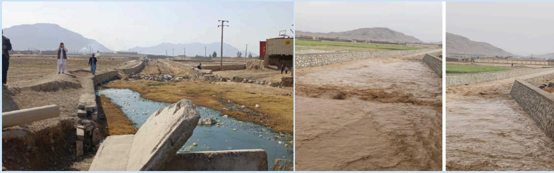
Construction of Norzai Canal Protection Wall with Total Length of 700m in Gozar #3, District #9, Kandahar City, April 2026
