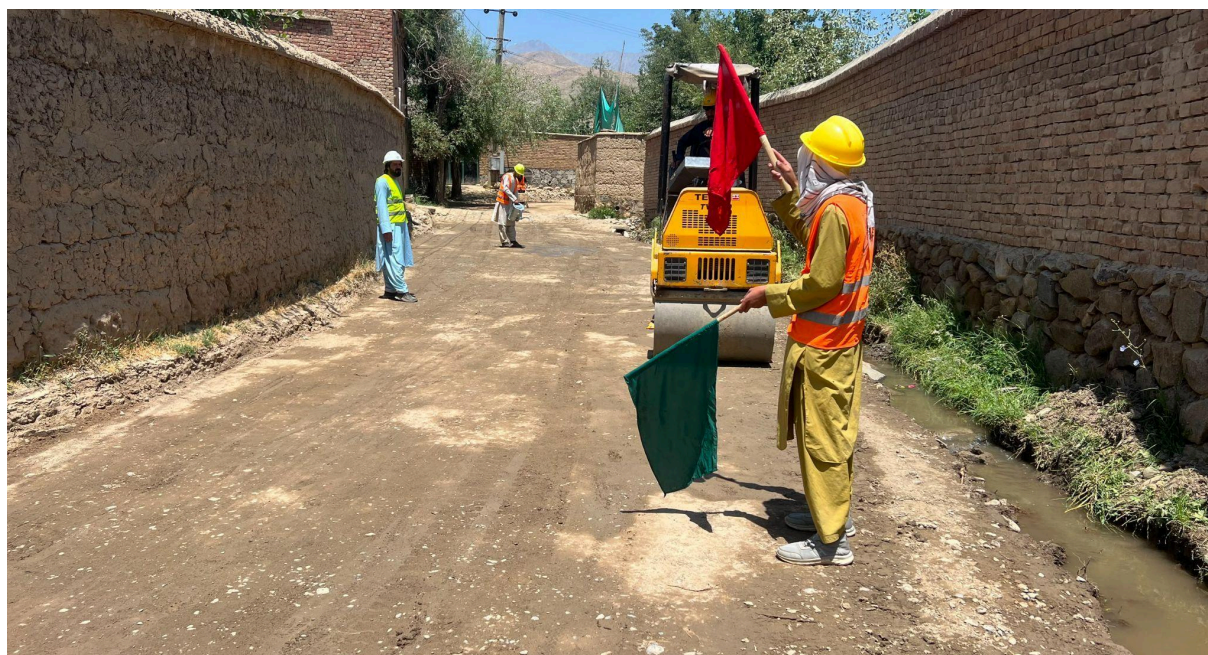
Subgrade compaction by roller machine in a LIW subproject in Kabul City, June 2026 @UNOPS
