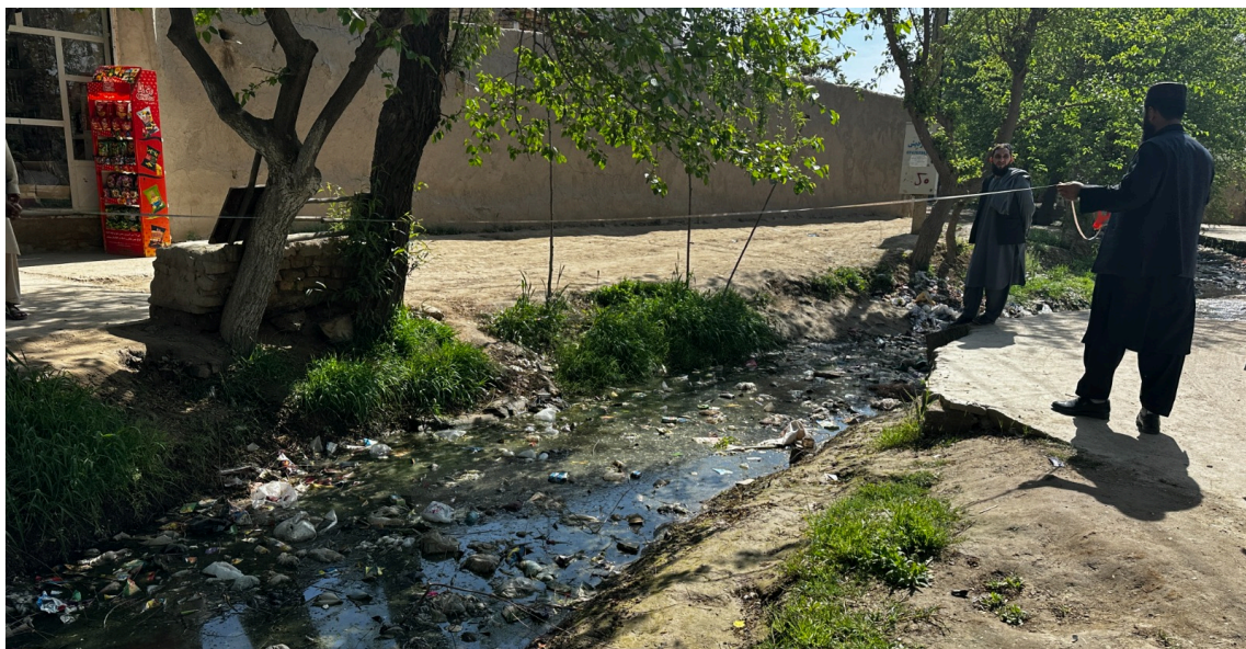
UNOPS Construction Management Engineers scoping for Construction of 220m Stone Masonry Protection wall for both sides of Canal Naqi Haiderqol, in Guzar 13, District 1 of Kunduz City. April 2026 @UNOPS
